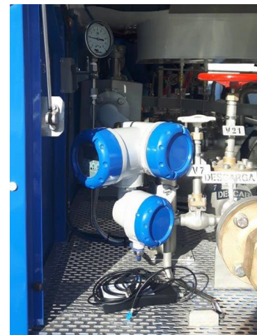
Converter of the OPTIMASS 6400 Coriolis mass flowmeter mounted on the LNG dispenser
