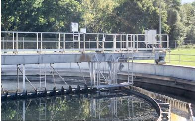
OPTISYS SLM 2100 and Radioline on the scraper bridge
