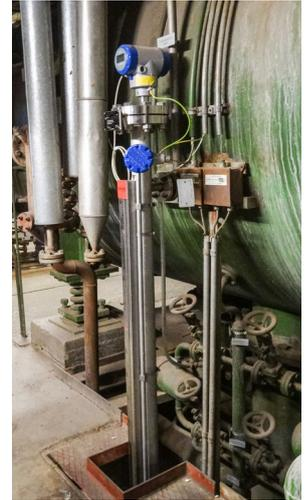
Bypass measurement with BM 26 A and OPTIFLEX 2200
