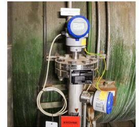
TDR radar signal converter (above) and LT40 electronics
