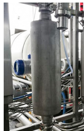
Flow measurement at raw milk reception with the OPTIMASS 1400
