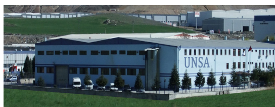
Ünsa Makina manufacturing plant
