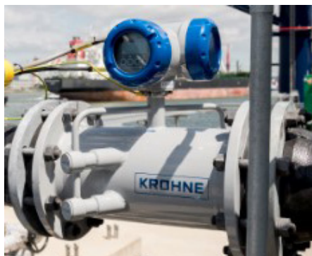
Ultrasonic flow measurement of hydrocarbon vapors
