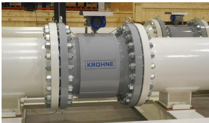
OPTIFLUX 2300 installed on water skid
