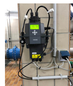
Online turbidity measurement with the OPTISYS TUR 1060
