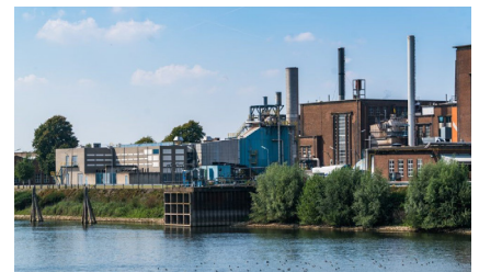
Historic boiler house with new biomass boiler in the Industrial Park Kleefse Waard (IPKW)
