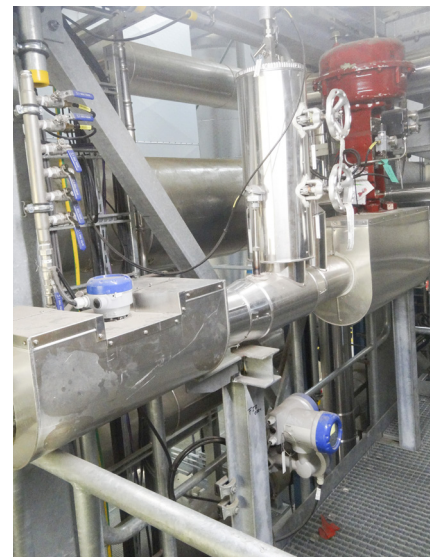
Feedwater measurement with the OPTISONIC 3400 ultrasonic flowmeter
