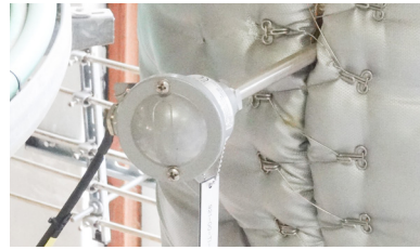
Temperature measurement with the OPTITEMP TRA-S34
