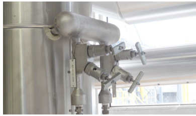
Venturi nozzle installation
