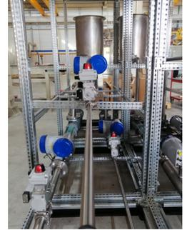
Dosing skid with EMF and Coriolis mass flowmeters
