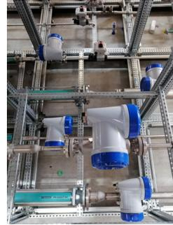
Flow measurement of additives for foam generation
