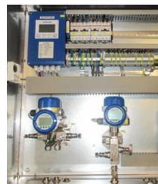
Control cabinet with KROHNE DP and pressure transmitters, temperature transmitter and flow computer
