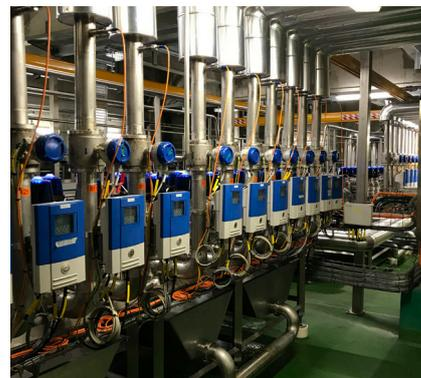
Flow measurement of beer with OPTIFLUX 6300 W (installed near beer tank)
