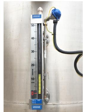
Condensate measurement with the BM26A-1000 magnetic level indicator and the LT40 reed-chain transmitter
