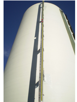
Level indication of treated effluent from uranium conversion
