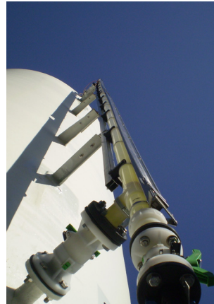
Magnetic level indicator tailored to 12 m / 39.4 ft tank height
