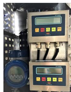
Field mount signal converter of the KROHNE Coriolis meter (left)
