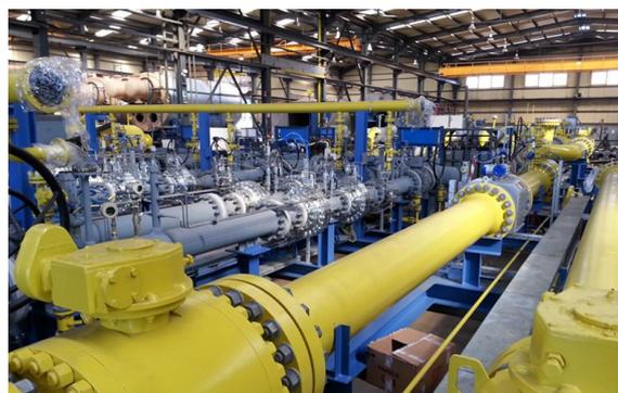
Fuel gas skid with ALTOSONIC V12 ultrasonic gas flowmeter
