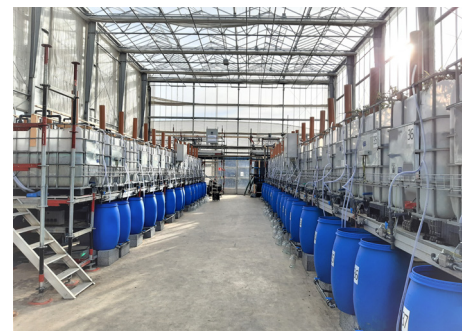
Test facility for sludge treatment and dewatering equipped with KROHNE flowmeters
