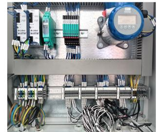
Remote converter of an OPTIFLEX 2200 level transmitter installed in a distributed I/O unit
