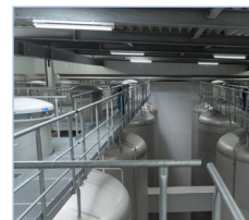
Pressure tank cellar with beer tanks
