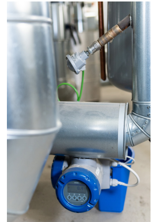
EMF with paired temperature sensor
