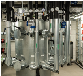
Concrete core temperature control
