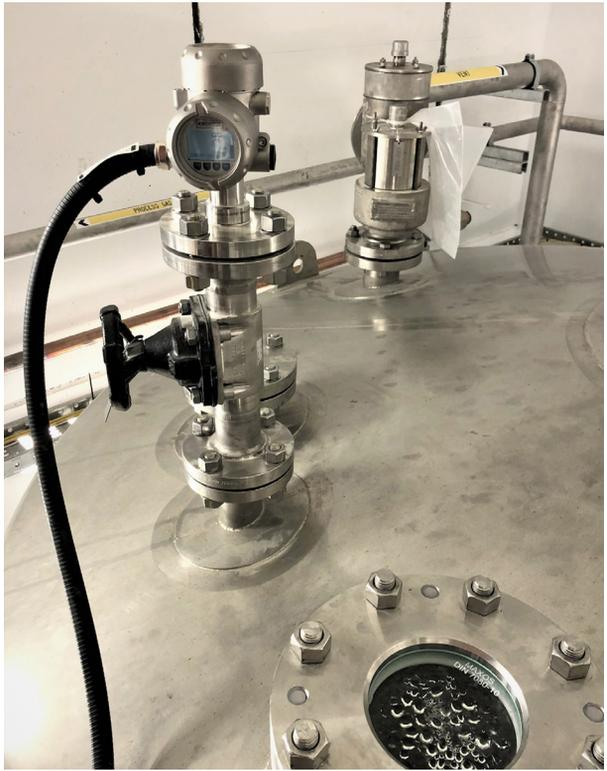
OPTIBAR PM 5060 for gauge pressure measurement in a tank
