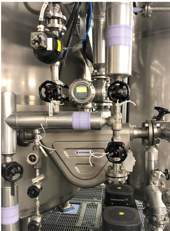
OPTIMASS 6400 measuring process condensate
