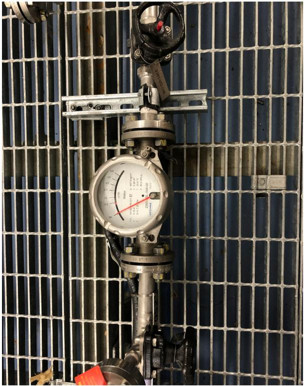
Water measurement with the H250 M40 variable area flowmeter
