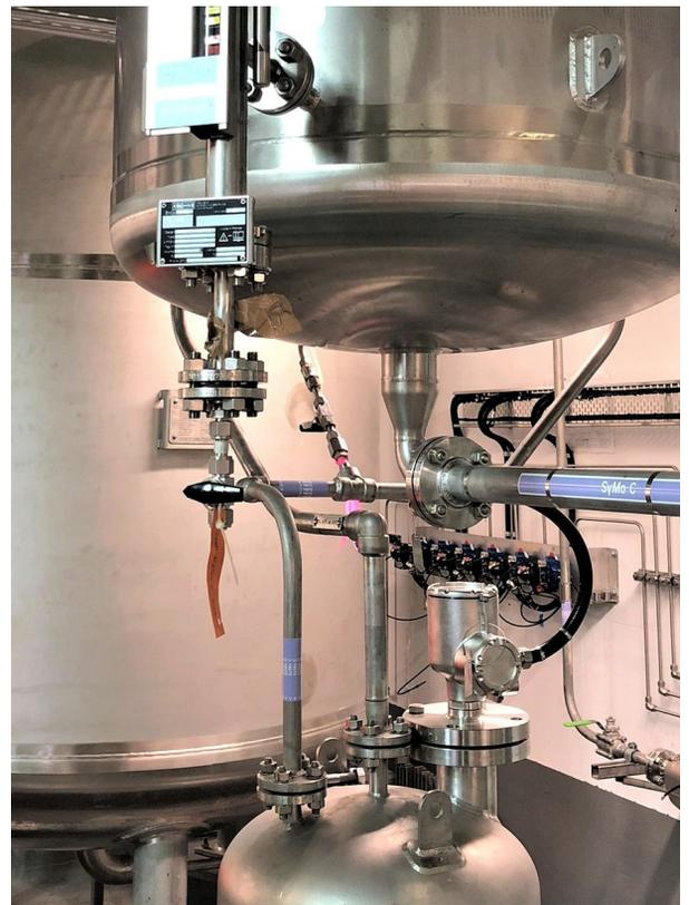
Level measurement on tanks using the BM26A-1000 level indicator and the OPTIWAVE 7500 radar level transmitter
