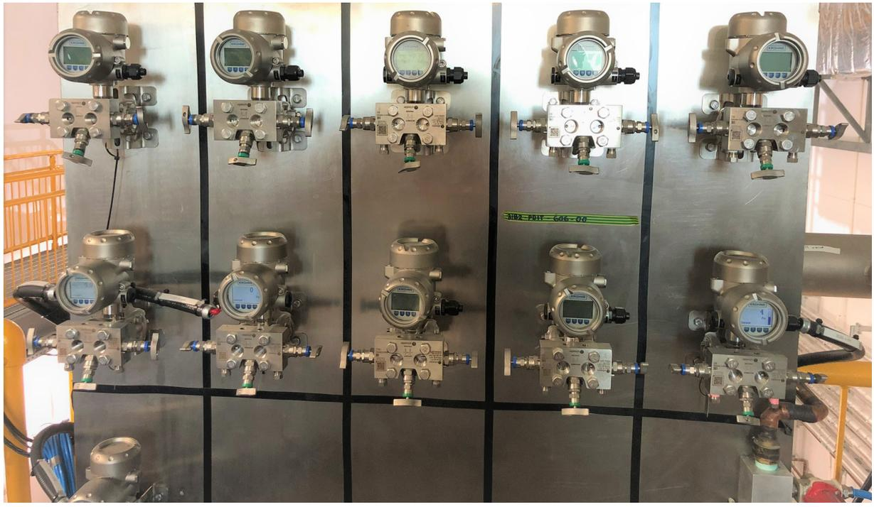
OPTIBAR DP 7060 used for hot cell pressure control and monitoring
