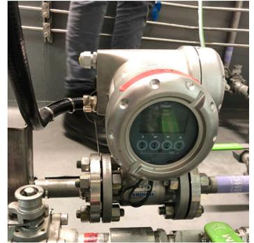
OPTIFLUX 5300 flowmeter for the chemical dosing of the special Synroc agent for treatment of waste from Mo-99 production
