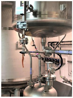
OPTIMASS 6400 measuring process condensate
