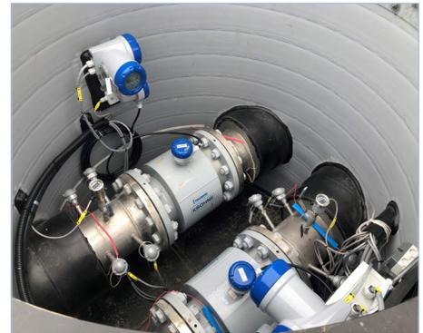
District heating measurement with OPTISONIC 3400 District Heating flowmeter, temperature sensors and OPTIBAR PM 3050 pressure transmitter
