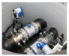
District heating measurement with OPTISONIC 3400 District Heating flowmeter, temperature sensors and OPTIBAR PM 3050 pressure transmitter
