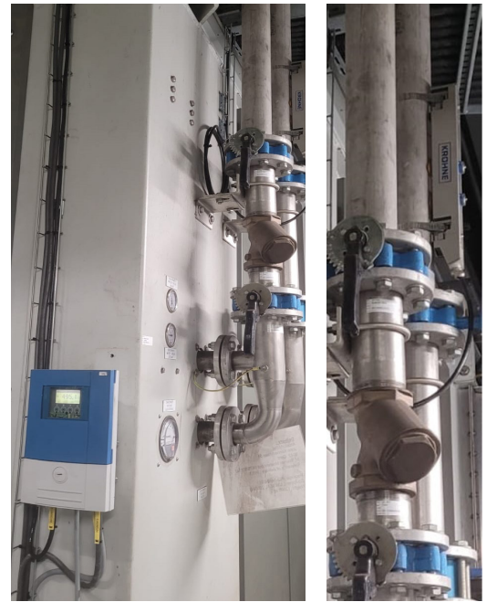
OPTISONIC 6300 with wall-mounted signal converter
