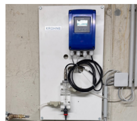
Water analysis panel with OPTISENS PH 8300 and integrated temperature measurement
