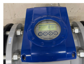
Flow measurement of laundry wastewater with OPTIFLUX 2050
