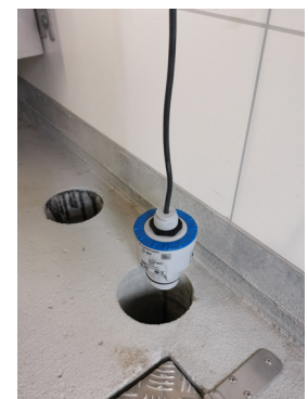
Installation of OPTIWAVE 1520 radar level transmitter
