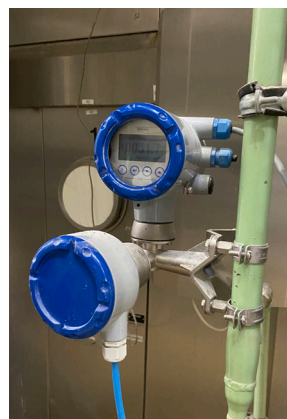
Field-mounted signal converter of the KROHNE Vortex flowmeter
