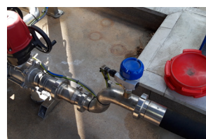
OPTISWITCH 5100 for dry-run prevention of pumps
