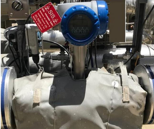
The flowmeters are available in sizes ranging from DN 08 to 250 and can be made in stainless steel 316L, Hastelloy® C22, and Duplex steel UNS S31803. The BASF installation includes 2-inch meters – the external meter is made of 316 stainless steel, while the internal is composed of Hastelloy.
